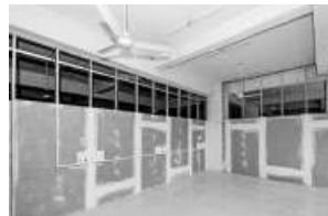
The newly-constructed 600-bed Covid hospital in Surat
